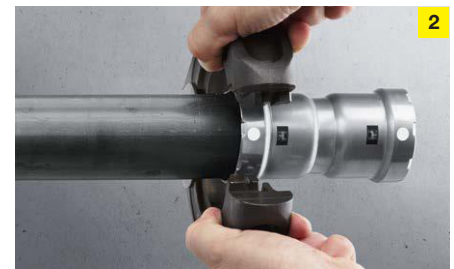
2 For pressing Megapress S connectors from 1 \frac{1}{4} inch upwards, only press rings with hinged adapter jaws are used. For smaller sizes between \frac{3}{8} and 1 inch, both press jaws and press rings with hinged adapter jaws are available.
