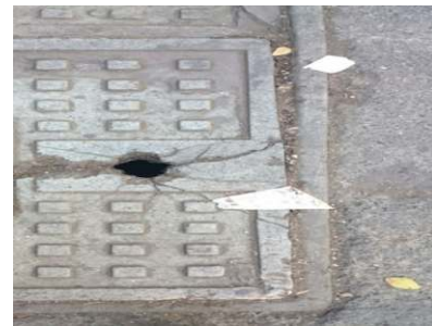
Condition of the Regular keyhole lifting arrangement of other make FRPmanhole covers
